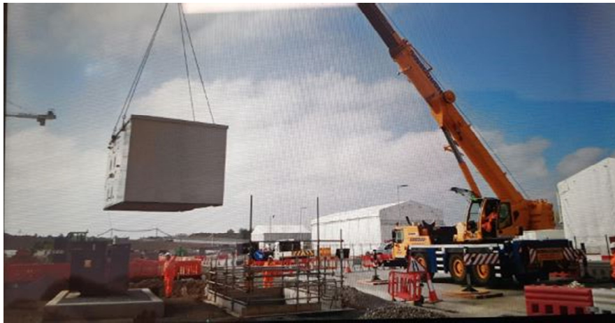
Figure 1: Work in progress during Hinkley Point C
