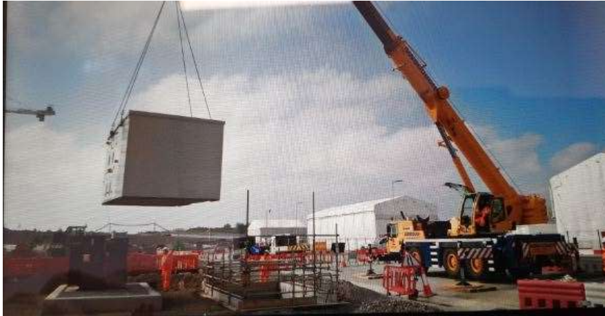
Figure 1: Work in progress during Hinkley Point C
